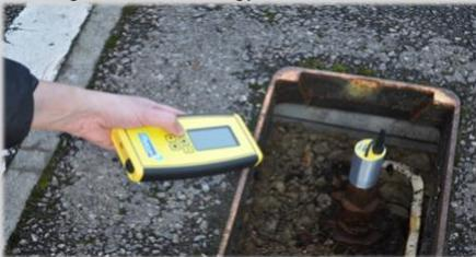
The loggers listen for any potential leakage. The data is retrieved and viewed daily, which can be easily downloaded to any PC for further analysis if required.
